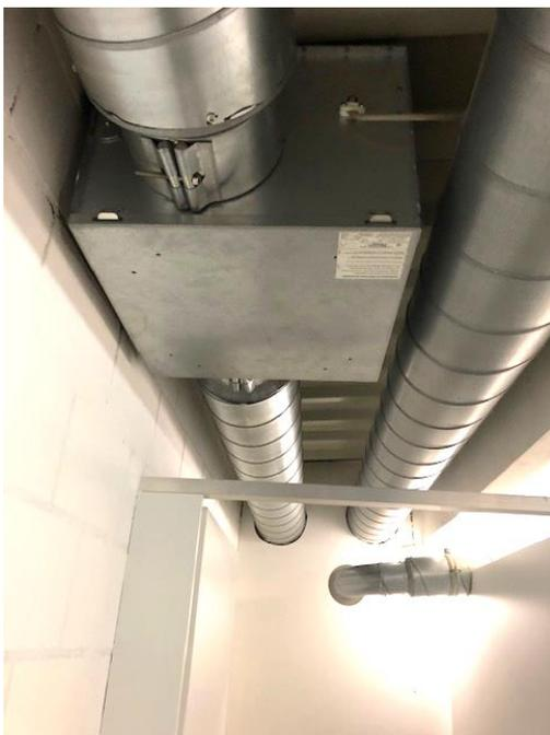
Abb. 41, Abluft Rohrventilator
